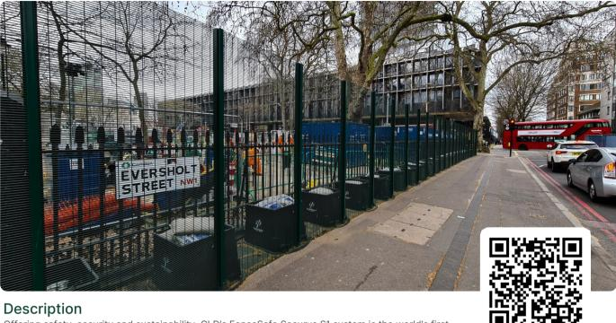
Offering safety, security and sustainability, CLD's FenceSafe Securus S1 system is the world's first LPS1175 security rated temporary fencing system. Using our innovative foundation free cantilevered FenceSafe base coupled with our Securus 358 mesh fencing, the system is guaranteed to offer at least 60 seconds delay against attack. Both the base and the Securus panels can be reused. The panels can even be used in a permanent fenceline.
